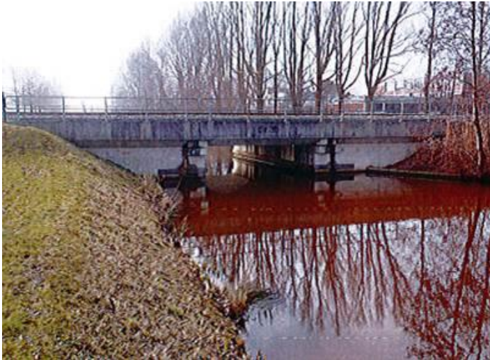
Betonnen spoorviaduct over water
