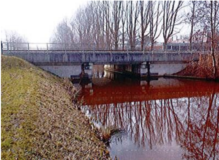
Betonnen spoorviaduct over water
