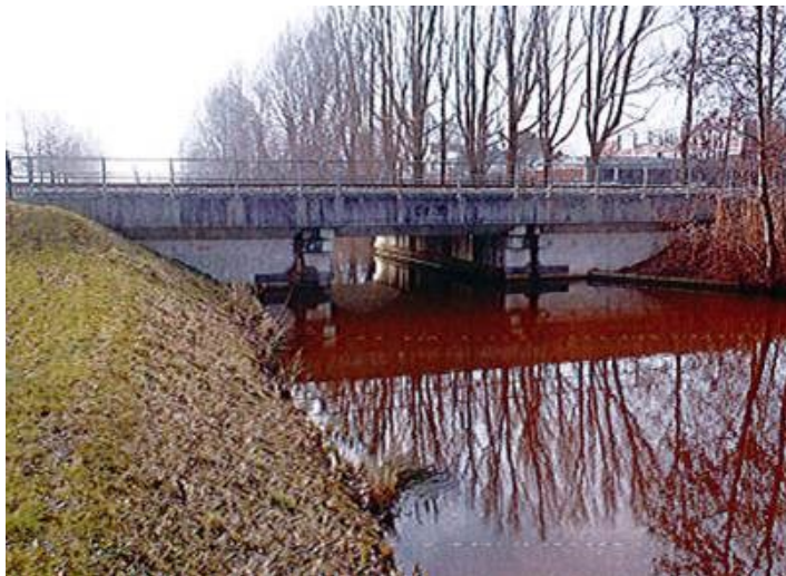
Betonnen spoorviaduct over water
