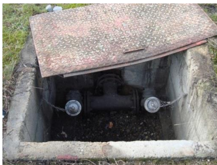
Bluswaterafnamehydrant
