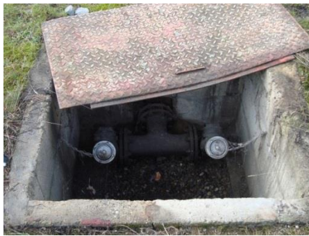
Bluswaterafnamehydrant
